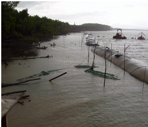
Sand-filled Geotextile tubes placed in front of eroding mangrove shoreline
