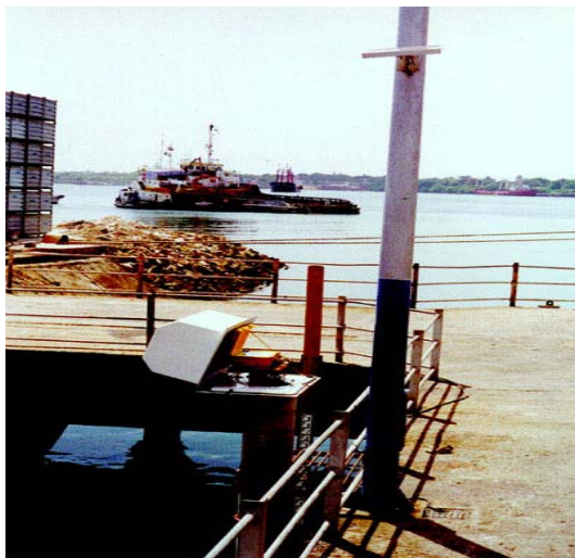
Tide gauge in Mombasa
